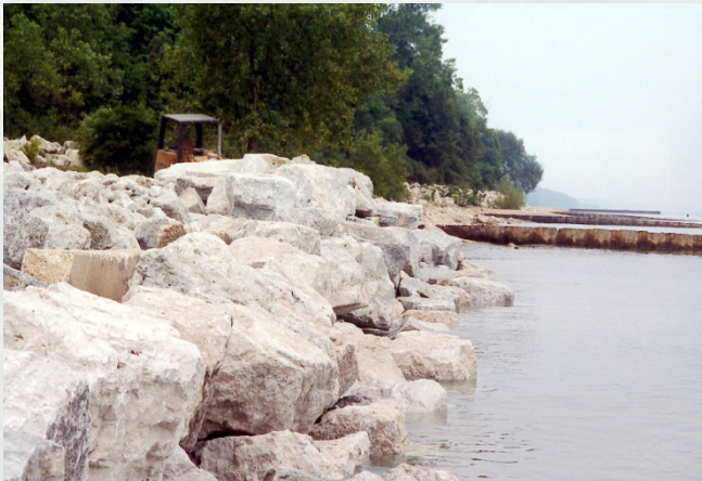
Construction and dredging Section 10 Rivers and Harbors Act
